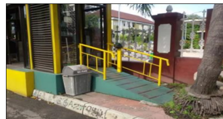
Figure 1. Ramp in Trans Jogja Shelter is Obstructed by Trees
